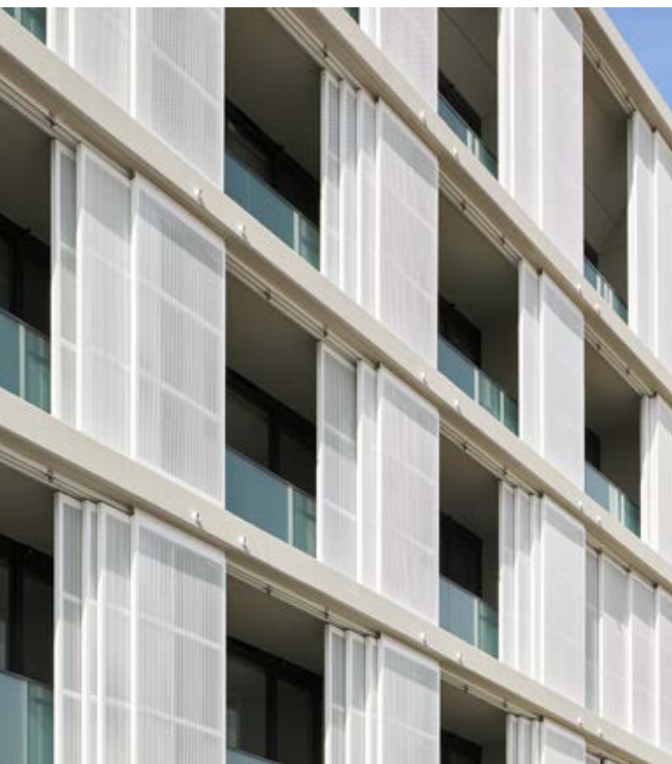
Sliding external shading helps to minimise heat from sunlight
